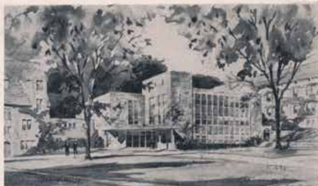
THE NEW UNIVERSITY STORE BUILDING
