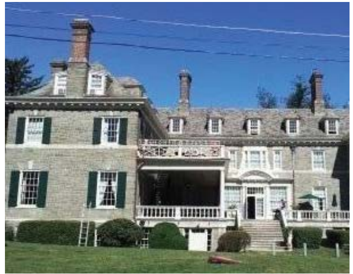
2013 summer renovation has corrected the porch balcony.
